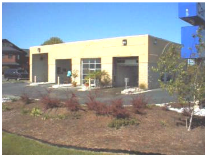
Carwash with vegetated area
